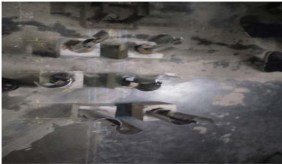
Fig. 6 : Cluster arrangement in double row
